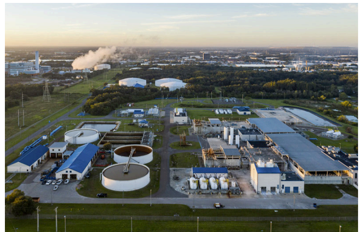
Tampa Bay Water's Surface Water Treatment Plant
