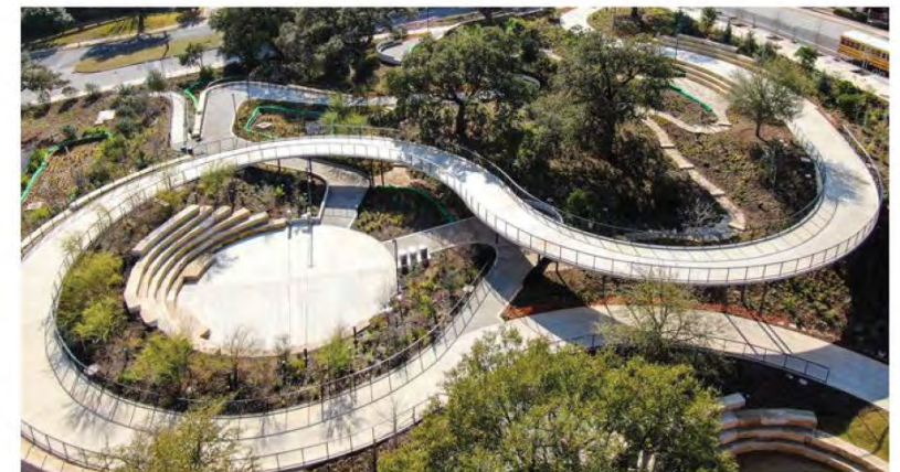
Waterloo Greenway Austin, TX
